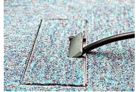
Steel lid topped by carpet
