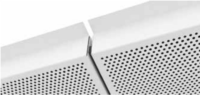
Gasket filled joint
