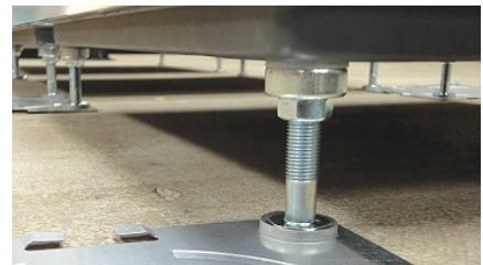
Step 1 and 3: loose and fasten the pedestal at the lock-nut at bottom
