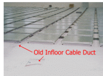
Renovation jobs: Installing on the old, embed floor trunkings
